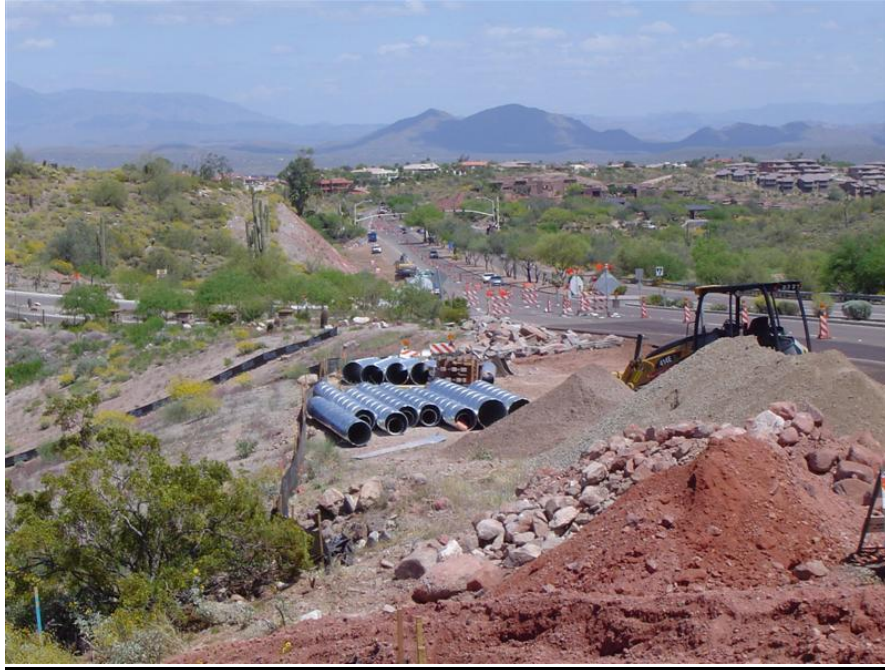
Shea Boulevard Construction – May 2011
